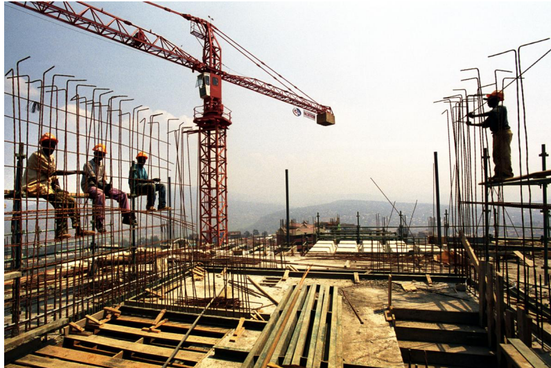
Construction in Kigali, Rwanda, August 2003 Sven Torfinn/ Panos Pictures / Redux
